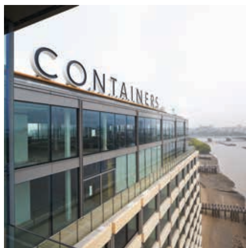
Above The lower three floors of the north facade were replaced with an aluminium cladding system, while two new office floors were added on the roof.
