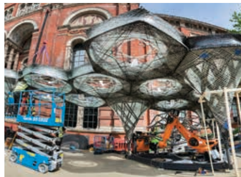
Above The pavilion's glass fibres act as a scaffold for the load-bearing carbon fibre structure. The weight of the 40 roof components is transferred to seven steel plates.
