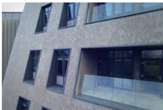
Left Corium brick cladding used on balcony and soffit areas.
