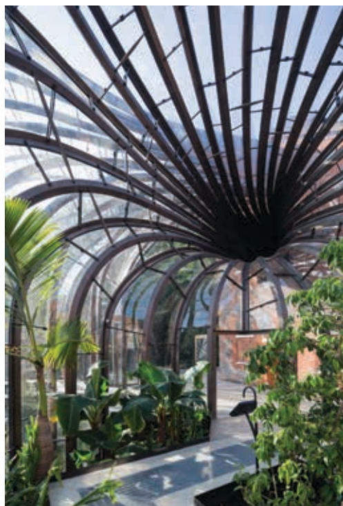
Above The geometry emphasises the flow of air through, up and away from the glass houses.
