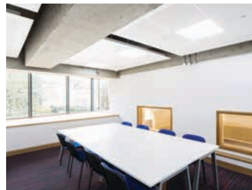
Above Armstrong Axiom Knife Edge canopy with ultra microperforated metal Tegular 2 tiles.
