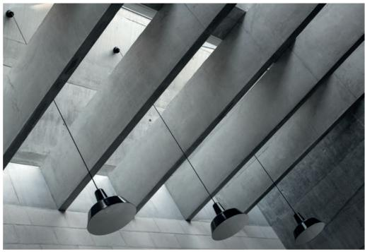
**Above** Concrete fin beams below the north facing rooflights of the studio space don't only look impressive, they act as baffles to deal with potential solar gain from east or west.
