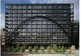
Left Detail of tied arch at SOM's Exchange House. steel structure.
