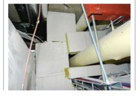
rated for 280 minutes for a 10mm by 10mm hole will only last 11 minutes on a 50mm by 50mm one. Use of the wrong PU foam is too common, often ignored or not identified, with a sample of inspections revealing an endemic problem. The message here was that PU foams do not replace a robustly designed and installed firestop approach.
