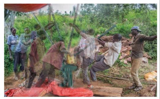
Jean Bosco compacts one earth block with the Makiga block machine, Ntarama, Rwanda, November 2014.
