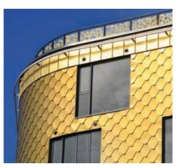
Installing one shingle at a time is a fairly labour intensive process which can result in higher labour costs when compared, for example, to running a 500mm-wide aluminium sheet from ridge to eave.
