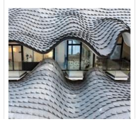
undulating amorphous roof punctured with complex curved window openings. A more crisp contemporary effect was achieved on the West Durrington Campus building at Northbrook College (see p.65) in Worthing, where NedZink NOVA zinc shingles continue around walls and soffits.
