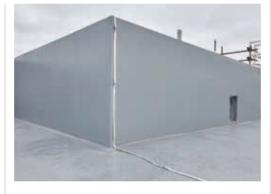
**Top** Visualisation of the completed school. **Above** Single ply was used to cover a storey-high change in roof height at Arnold Hill, removing the need for a render finish.
