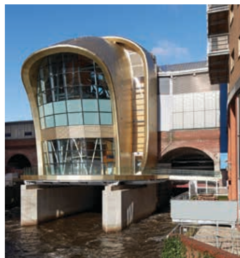
Left Passengers have views of the exposed diagrid steel structure as well as the River Aire as they travel on the escalators.
