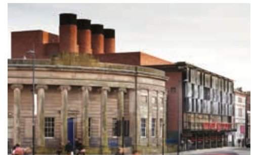
Above Everyman Theatre's chimneys have to generate adequate buoyancy to pull sufficient fresh air through to keep the auditorium comfortable
