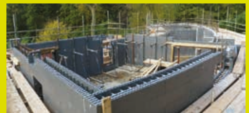
Curved Thermowall Construction
