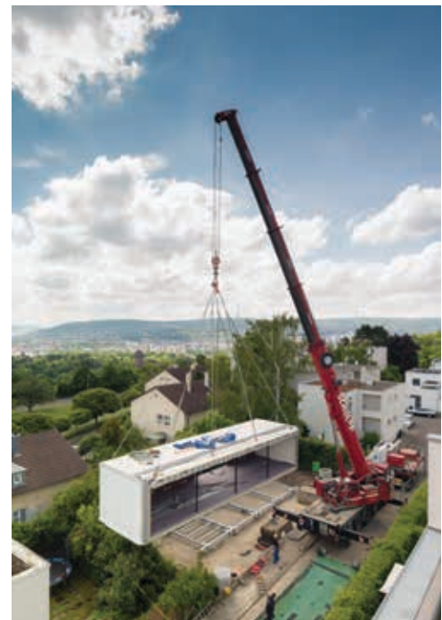
Above The living unit, one of two prefabricated volumes forming the Aktivhaus, being craned onto site.
