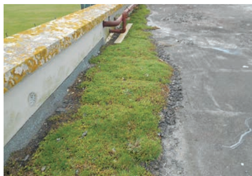
Top Temperature variations between ponded and dry areas can result in cracking.
