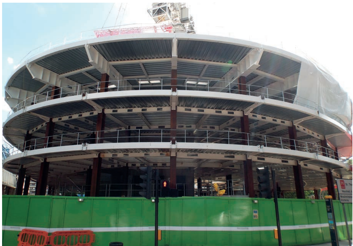
Above The radial steel structure of the sixth form college at the base of the tower.
