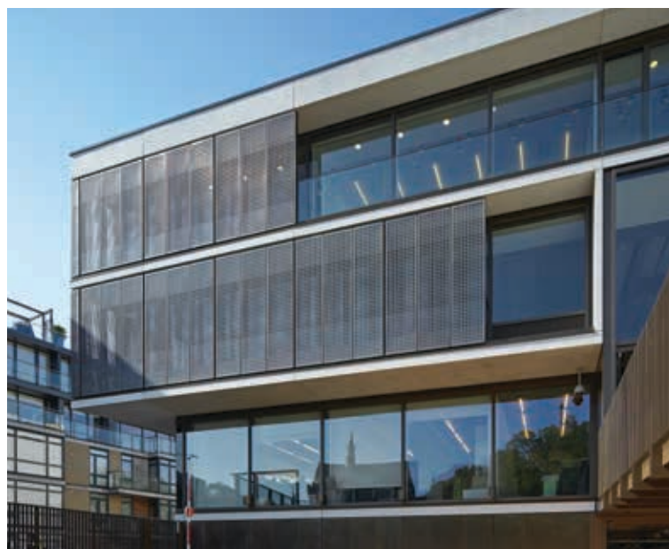
Above JW3's main pavilion elevation was designed to be highly blast resistant. Left Pavilion detail showing perforated bronze shading panels.
