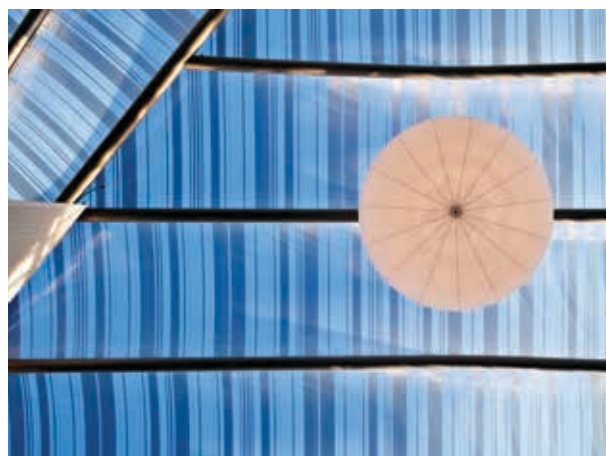
Top Detail of the precast panels which create a play of light and shadow, their depth also ensuring a layer of solar shading internally.
