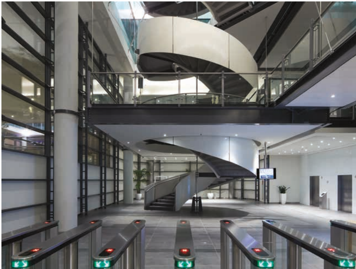
Left The stainless steel stair and lobby walkways are hung from Macalloy bars, getting the minimum amount of material to work hardest in tension.
