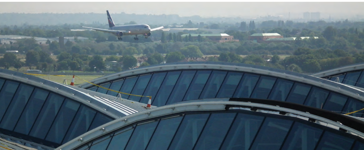
Left The new terminal's distinctive undulating roof incorporates approximately 7,000m 2 of Schueco's framed glazed skylights.
