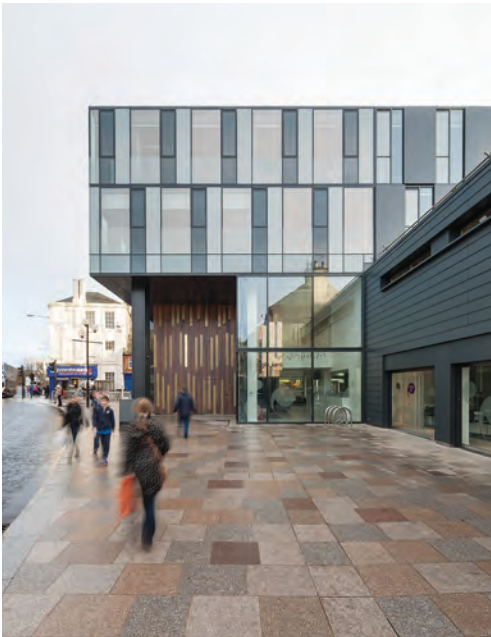
Left Before and after of the façade with single glazing replaced by a Schueco structural glazing system.
