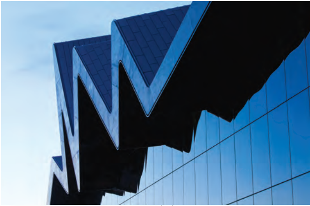
Far left Unitised structural glazing creates gable elevations rising 19.8m including some highly irregular panel sizes (left) .
