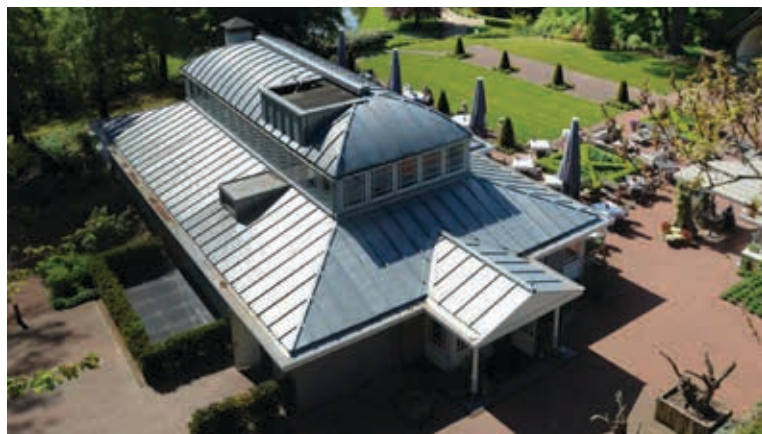
An example of natural zinc sheet roofing brings a crisp finish to roof detailing.
