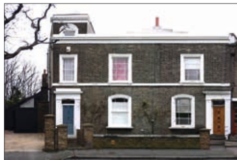
ABOVE: The end-of-terrace Priory Grove house – and its neighbour – 40 years ago and (right) as it is today. Extensions to the top and left hand side of the building have repositioned the main entrance at the centre of the now double-fronted home.
