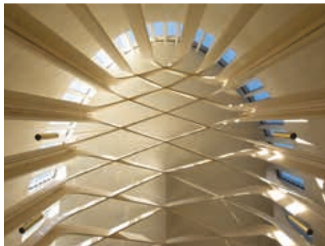
The protruding niches are left over from the removal of the elliptical plan's original enclosing box. BELOW: McLaughlin's fine timber structure appears to hold the roof down rather than up.
