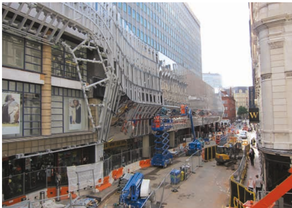
Left The north facade of Birmingham New St station receiving its mirrored stainless steel appliqué on a secondary steel structure attached directly to the existing concrete structure.
