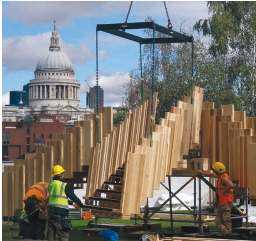
Clockwise from top left Visitors explore Endless Stair; installation outside Tate Modern; corner section of the stair showing the CLT boards; components were largely constructed off site; the timber has a warm and textured finish.
