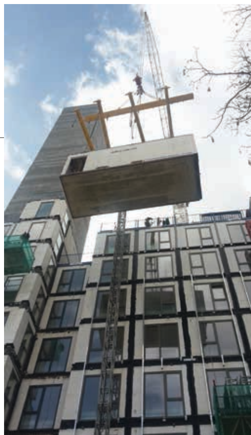
Modules being placed at a rate of 10 a day at Apex House in Wembley, London.
