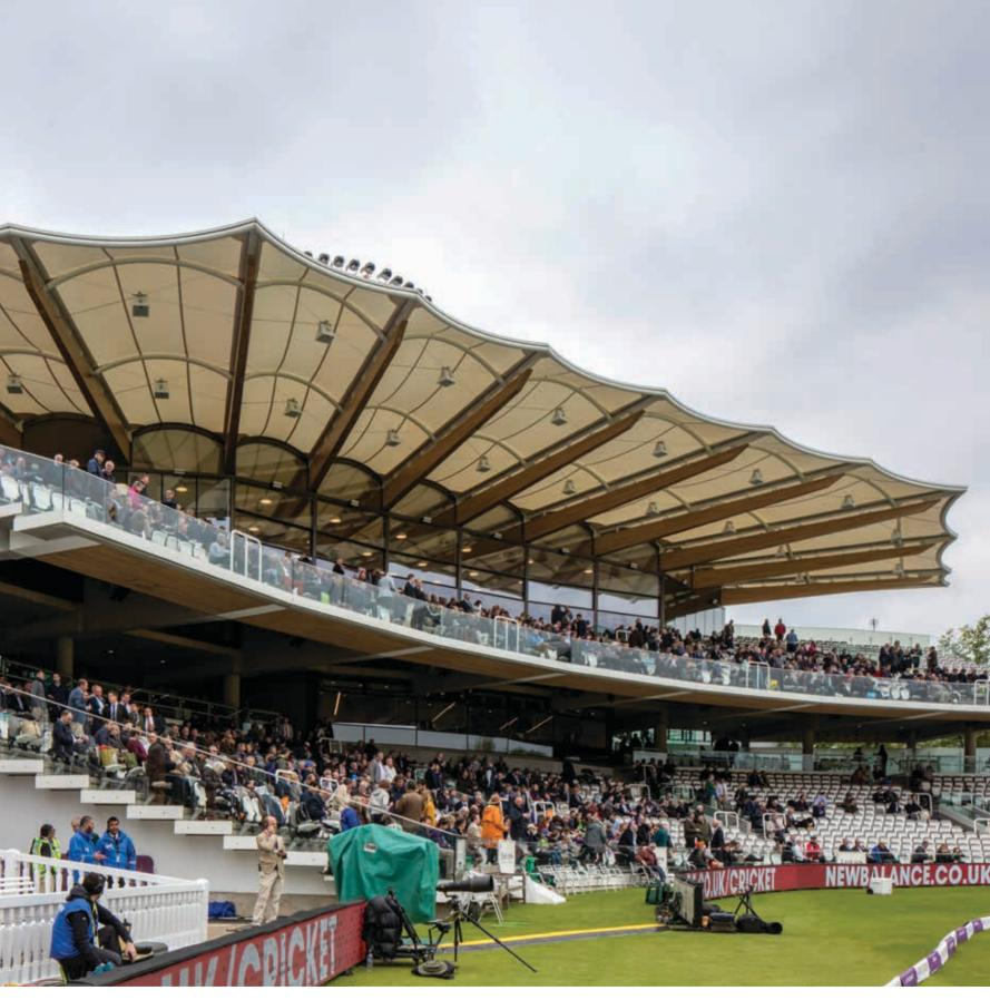
**Above** At the opening match the view into the Warner Stand from the pitch shows the simple continuity of what is apparently a single roof when seen from below. **Right** The top tier in the Warner Stand sits under a thin stretched fabric skin.
