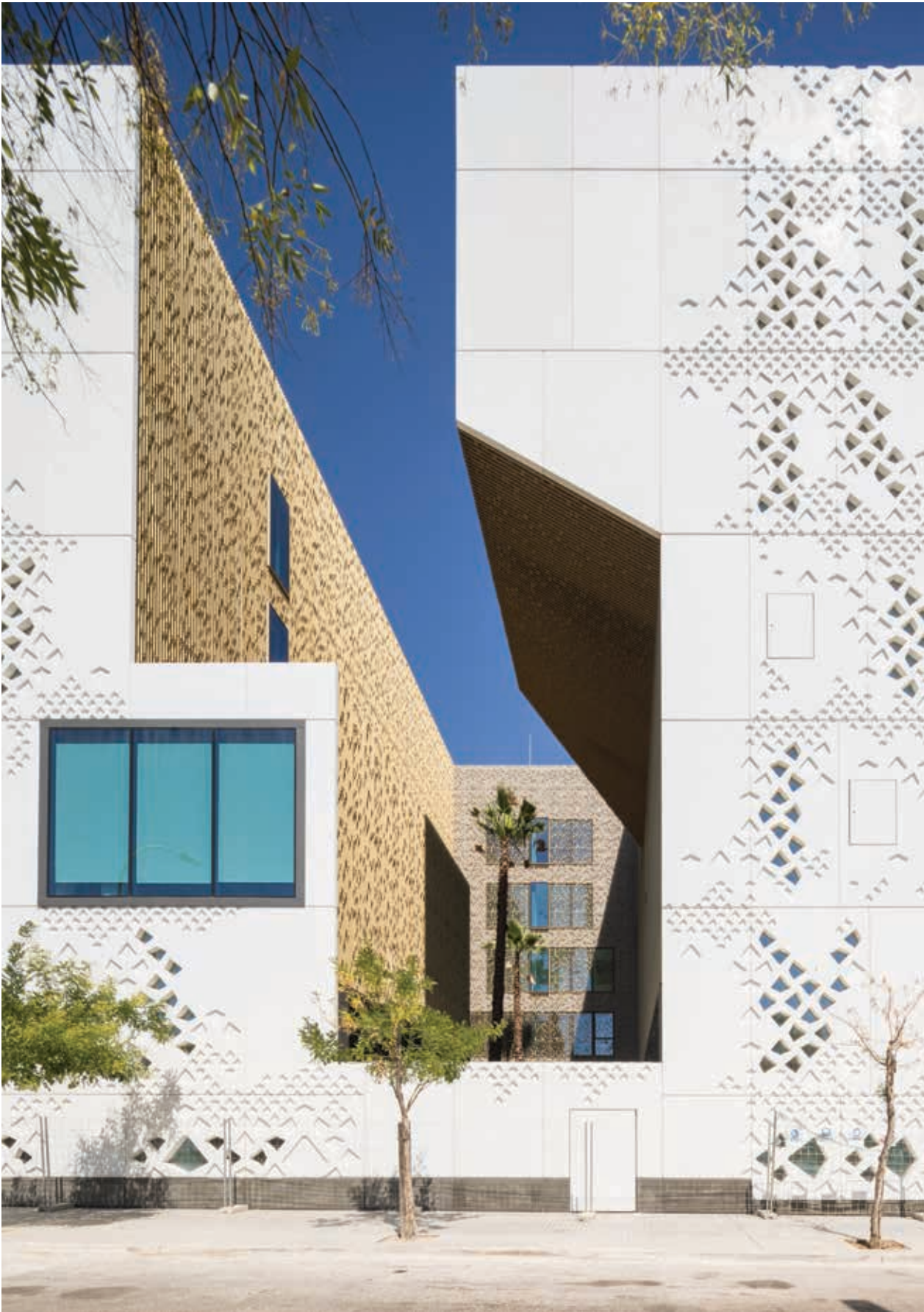
Right Gold anodised aluminium latticework covers the surfaces that have been exposed in the carving out of the massive GRC facade.
