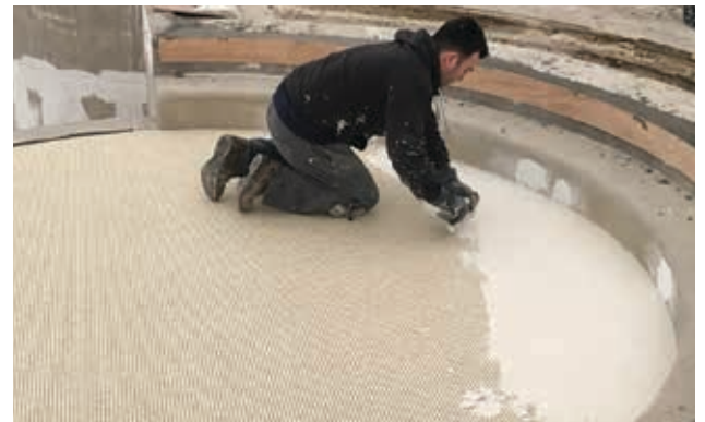
Right Grouting the mosaics on the pool floor with Fugalite Bio Ivory.
