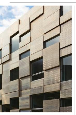
aluminium folded rain screen cladding panels, which stagger 100, 150 or 200mm from the insulation line, generate a layered, staccato effect that picks up the soft Bergen light differently every day. With folds each set at the same angle, it creates further facade modulation by varying the size of the shadow gap between cassettes. But the 0.04 U-value is created via 250mm of Rockwool and 500mm aluminium sandwich panel behind it.
