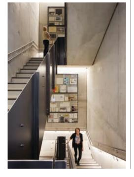
Left With exposed concrete cores and floors, thermal mass principles are employed in the structure.
