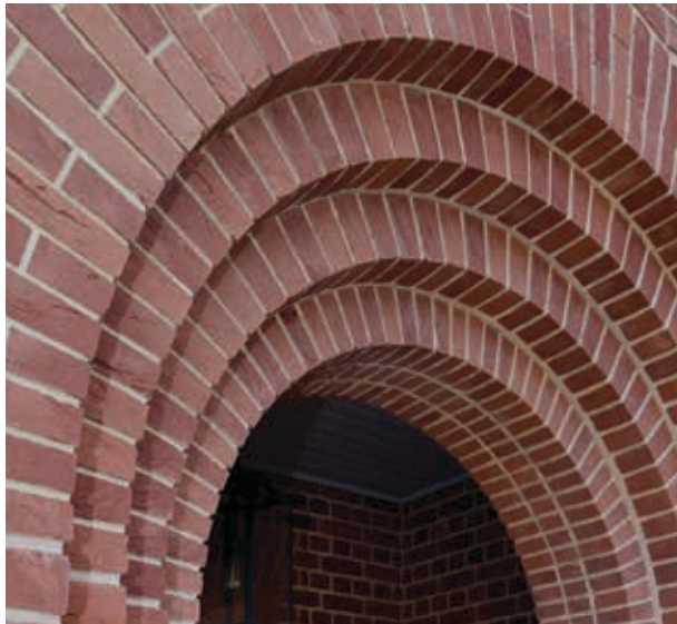
Above left The Queens Wharf project featured IG's B.O.S.S. system to achieve the stepped brick element over the openings.
