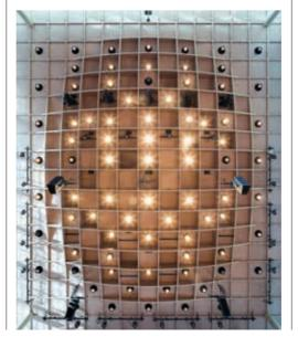
the CNC-cut beech LVL acoustic grid and the inset clerestory also add a sense of enclosure.
