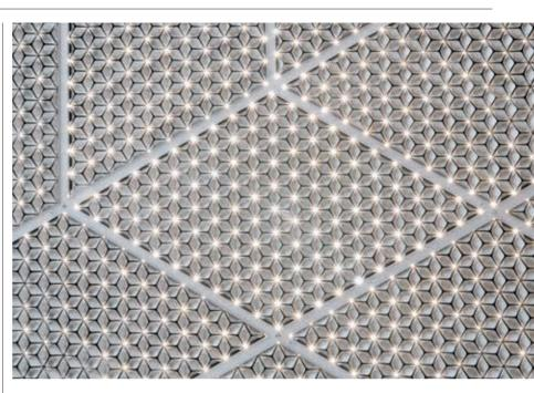
Above Detail showing the 2.5 million aluminium petals that make up the ceiling for cooling, acoustics and lighting.
