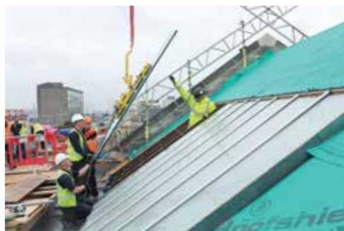
Left Installing the glass on one of the rooftop studios.
