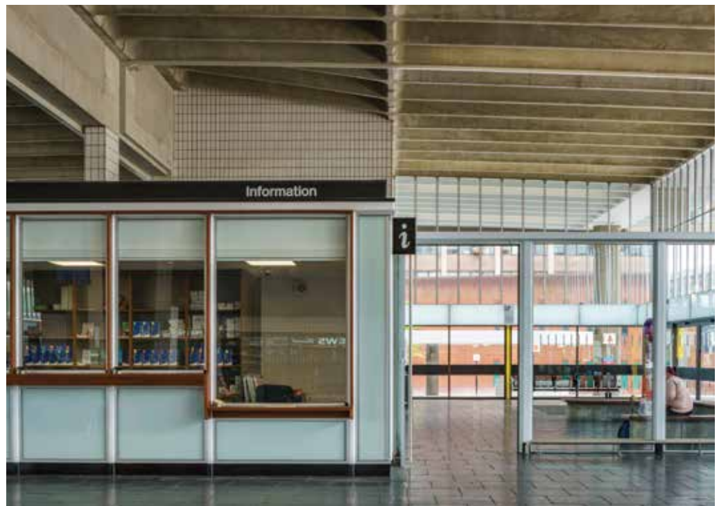
Above Insertions such as the reception pod use the lighter language of steel and glass but also repurpose the original iroko barrier boards.
