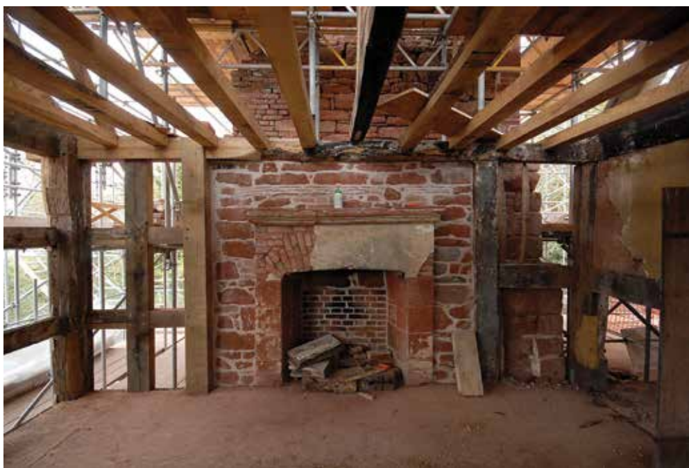
Above Timber beams, old and new, starting to be put back into place.
