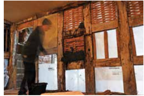
Right Wattle and daub being applied to new lath structure.
