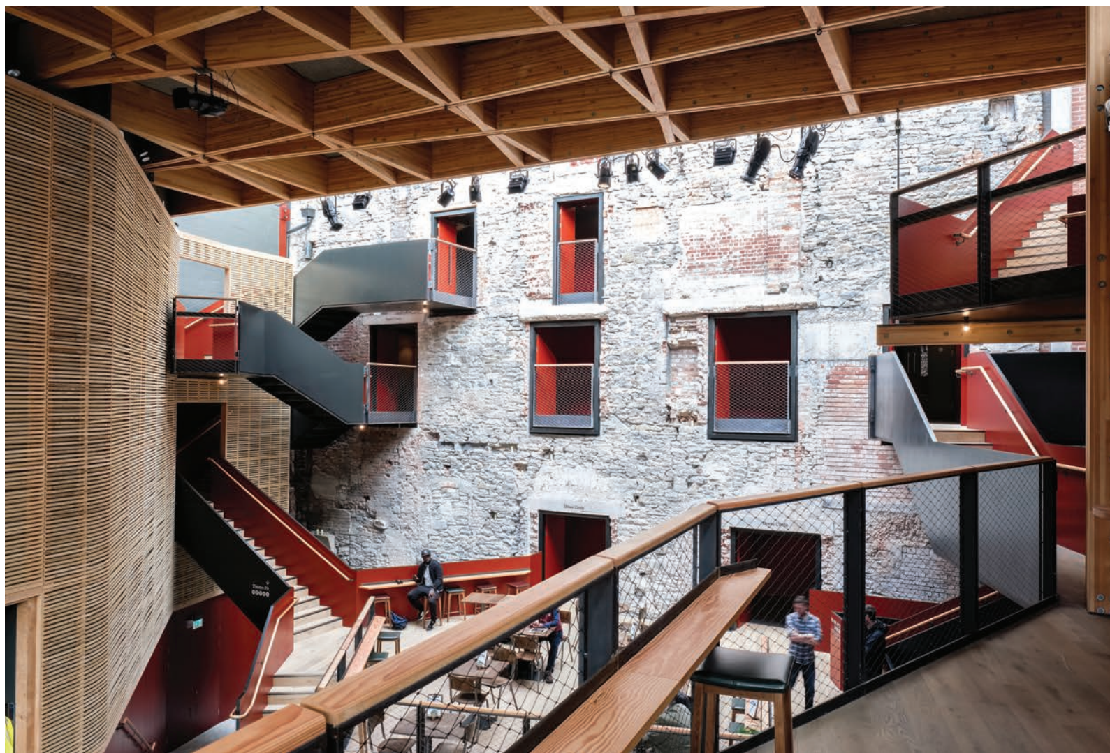
Above The glulam frame of the foyer against the masonry fragments of history.
