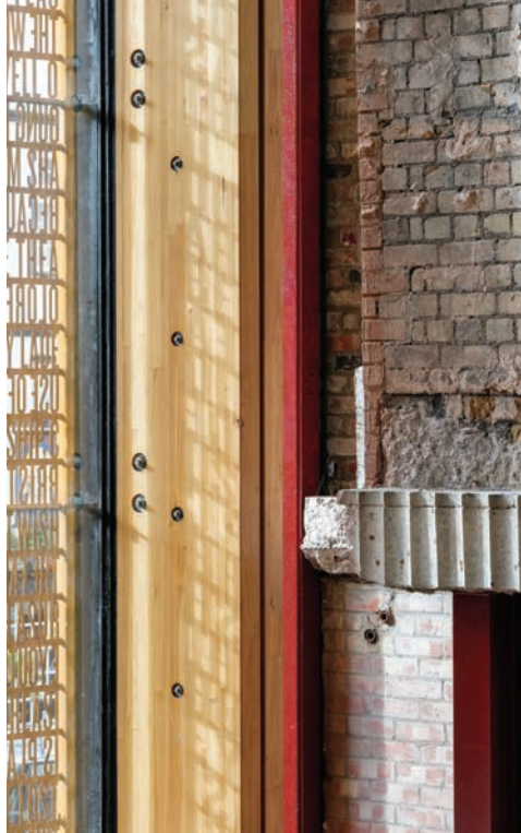
Above The glulam frame of the foyer against the masonry fragments of history.
