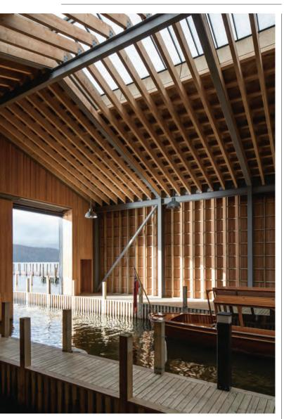
**Above** It was almost inevitable a boathouse would be central to the design. The large sliding doors are 5.6m high and 4.3m wide to allow boats in and out of the museum.
