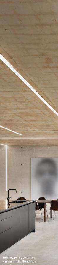
This image The structure was cast in situ. To achieve the column-free living space here 70 tonnes of steel were required.
