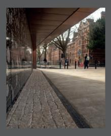
As the different academic roles interrelate inside, so must the various components that are employed to protect the building envelope and the external access routes. Swiftly removing surface water from the surrounding path and cycle ways, ACO's MultiDrain MD is reliably efficient. Classically designed ductile iron gratings fit securely to the channels, complementing the heritage setting.
