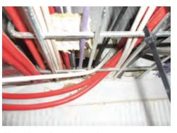
Above Missing fire stopping in fire compartmentation found in recently constructed public buildings in Scotland.
