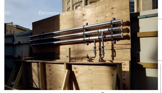
**Above** Visualisation of abbey without pews. **Left** A full-scale mock-up of the pipework system and Great Drain constructed outside the abbey.
