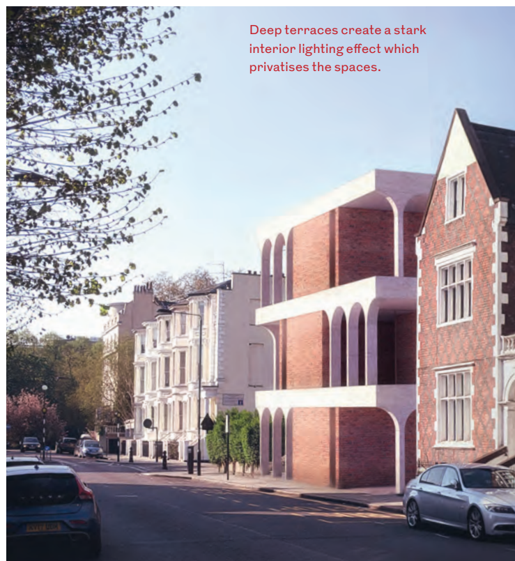
IG Lintels brick slip soffit solution around the perimeter edge enabled a floating upper storey.
