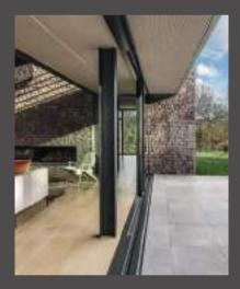
Silver How could have been just another house, but, as Wainwright afforded the mountain it's own chapter, the Arts and Crafts period stable has its own story. Simple ACO Brickslot gratings remove surface water along the discreet, level threshold which has been opened up with new glazing bringing the courtyard into a house developed with detail in mind.
