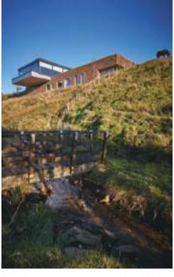
Above The balcony was a late addition to the end of glass box and caused the cantilever structure to get thicker, visible by the lighter grey cladding.
