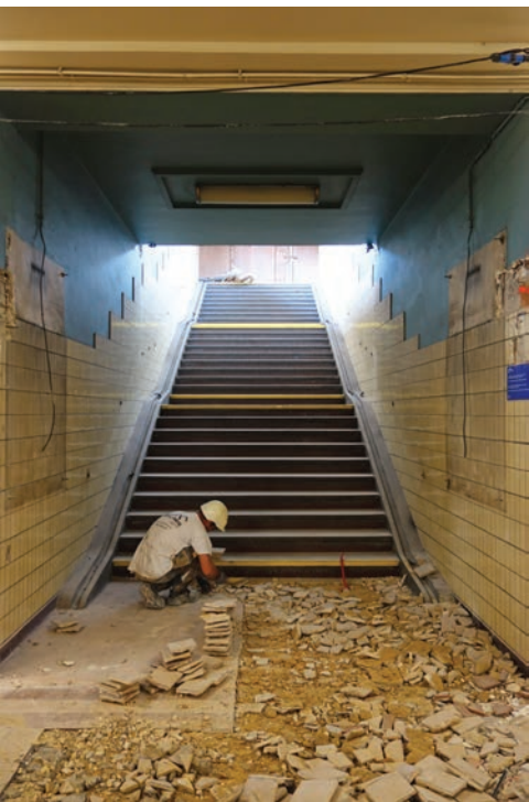
Above Belgian firm Rotor carefully removing materials to allow them to be re-used on other projects.
