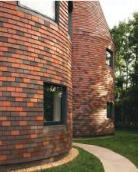
Below The house is entirely clad in ceramic tiles, changing from darker at the bottom to lighter at the top.
