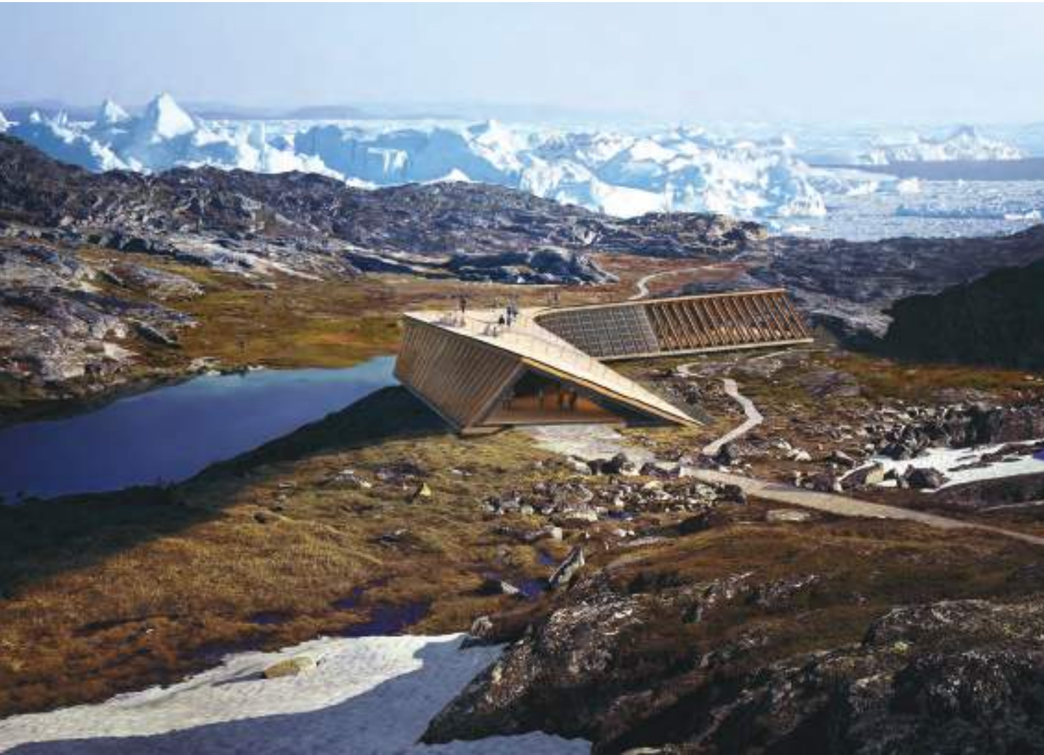
Below Render of the Icefjord Centre, Ilulissat, Greenland, currently on site 250km north of the Arctic Circle. Its section twists so the roof can also be used as a viewing platform. This and the boomerang plan reduce the snow load by shedding it.
