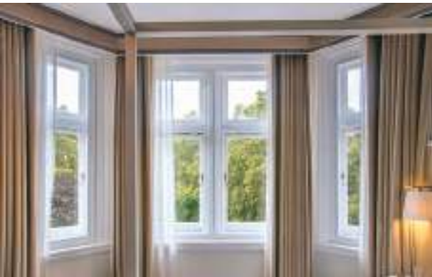
Left Granada Glazing’s horizontal sliders are both slimline and discreet, they match the style and function of traditional casement windows. The panels can be lifted out of the frame to give full access to clean the primary windows. This is often a consideration missed when working on hotel projects or projects that require frequent access for cleaning and ventilation .
