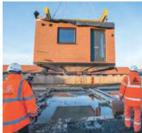
Above Modules on the production line at the Ilke Homes factory in Knaresborough, North Yorkshire: safer, quicker, cleaner, more sustainable. Left Architecture as product design: a module being craned into Ilke Homes' Hawthorne Avenue development in Hull.
