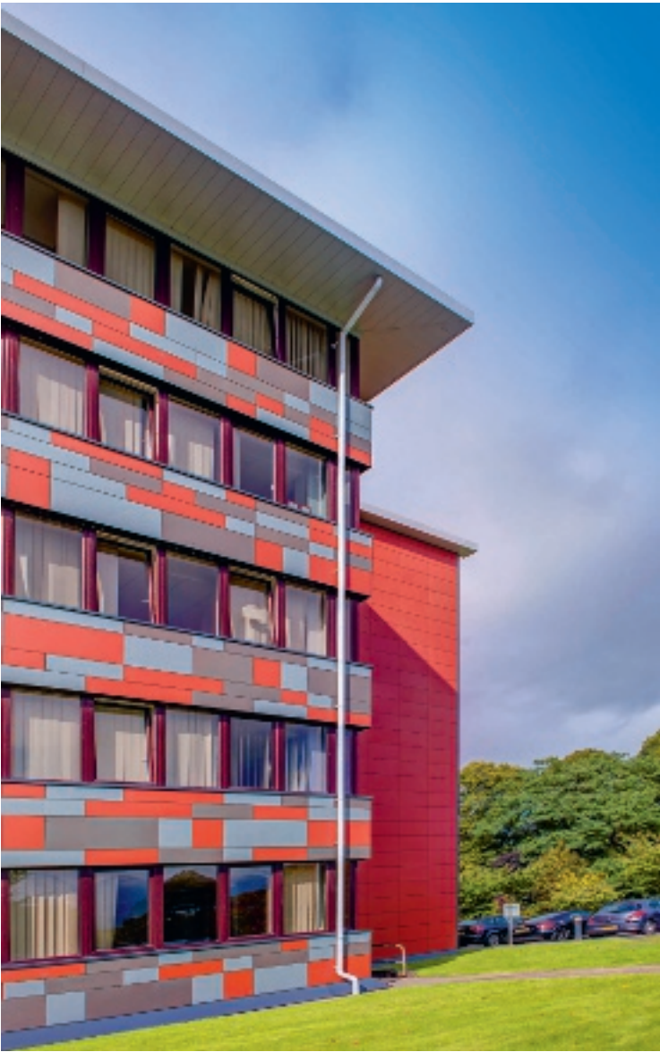
Left Equitone Natura panels can be cut and arranged in horizontal, vertical and angled layouts.
