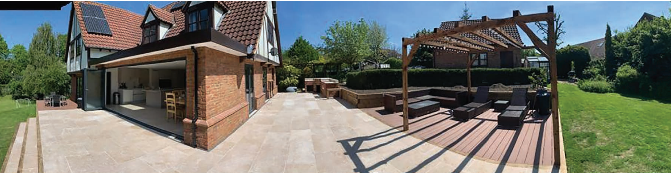
Above The limestone tiles have been laid over the Green-Pro membrane to ensure a trouble free installation. Left Biogel No Limits and Fugabella Color were used to fix the tiles over the underfloor heating in the kitchen.
