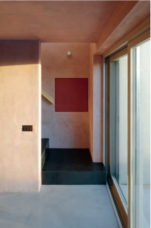
Left Clay plaster, polished concrete floor, steel stair, wood handrail and window frame make a composition of colours and textures.
