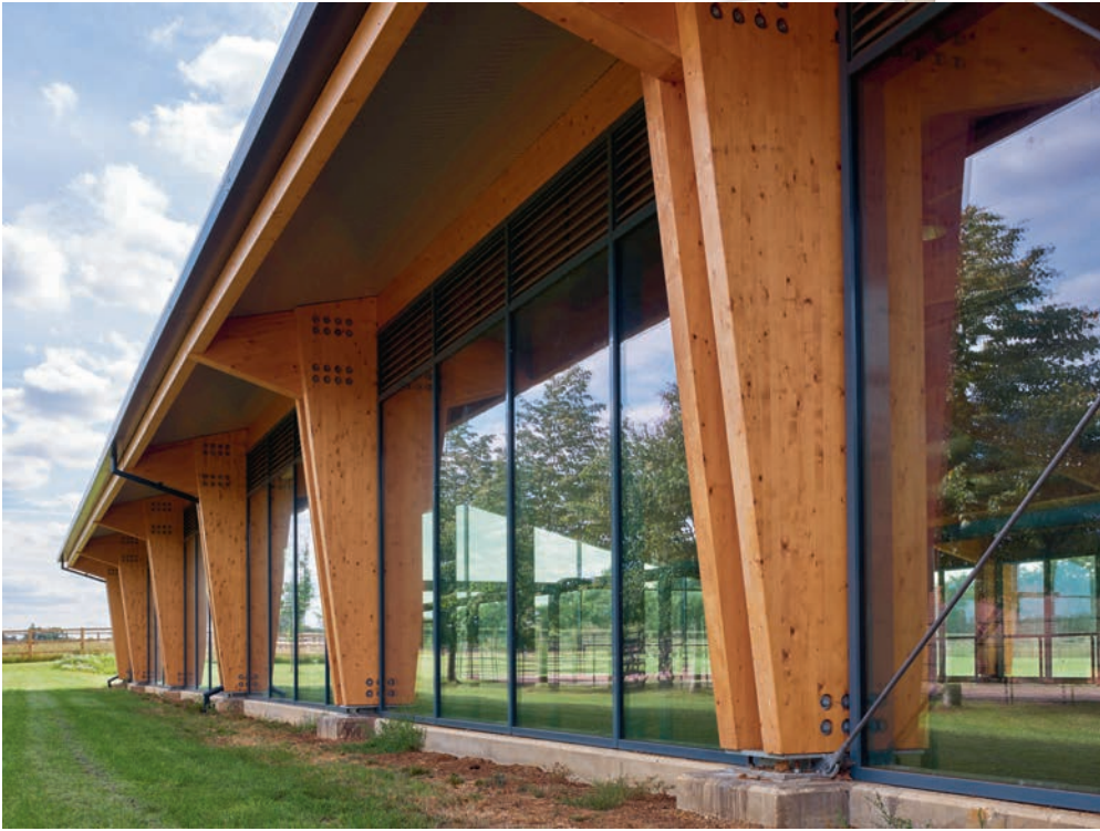
Below The overhanging and well insulated roof ensure the manège stays cool.
