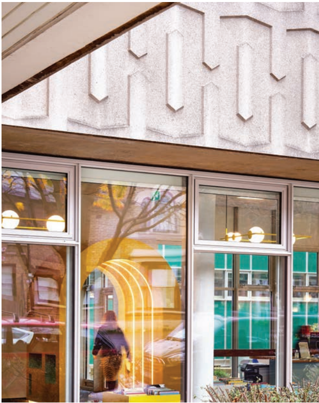
Left Spalling on the original patterned concrete exterior has been left so resources could be prioritised on improving the performance of the roof and other parts.
