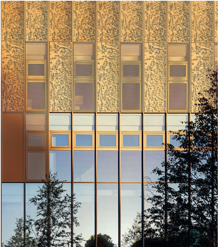
Above and right Facades are composed of concrete panels interspersed with perforated anodised aluminium ventilation panels. 'The warm hues and natural tones of the materials play well with the changing quality of light throughout the day and the seasons, discretely animating the facades', suggests the architect.
