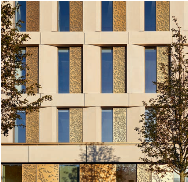
Above and right Facades are composed of concrete panels interspersed with perforated anodised aluminium ventilation panels. 'The warm hues and natural tones of the materials play well with the changing quality of light throughout the day and the seasons, discretely animating the facades', suggests the architect.
