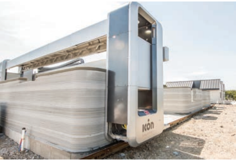
Right Vulcan takes 24 hours to print 400-500ft² of wall, spread across several days.
