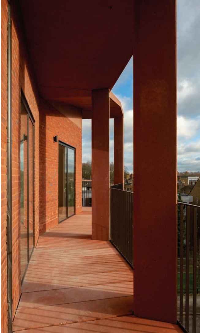
Left Brick walls bear on precast balconies at Wilmott Court. Right Triangular loggia columns at Wilmott Court avoid shaded inner faces.
