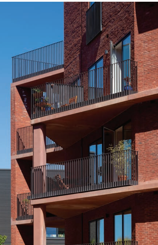
Left Brick walls bear on precast balconies at Wilmott Court. Right Triangular loggia columns at Wilmott Court avoid shaded inner faces.
