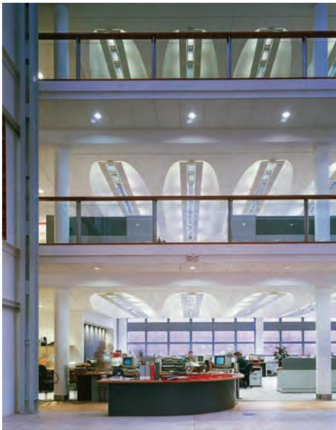
An exposed vaulted slab helped thermal cooling at the PowerGen HQ – one of the marginal gains that gave it the edge.
