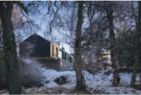
Right and left The new extension continues the ground floor of the original farmhouse over the sloping side onto a new plinth that ends with a cantilever.
