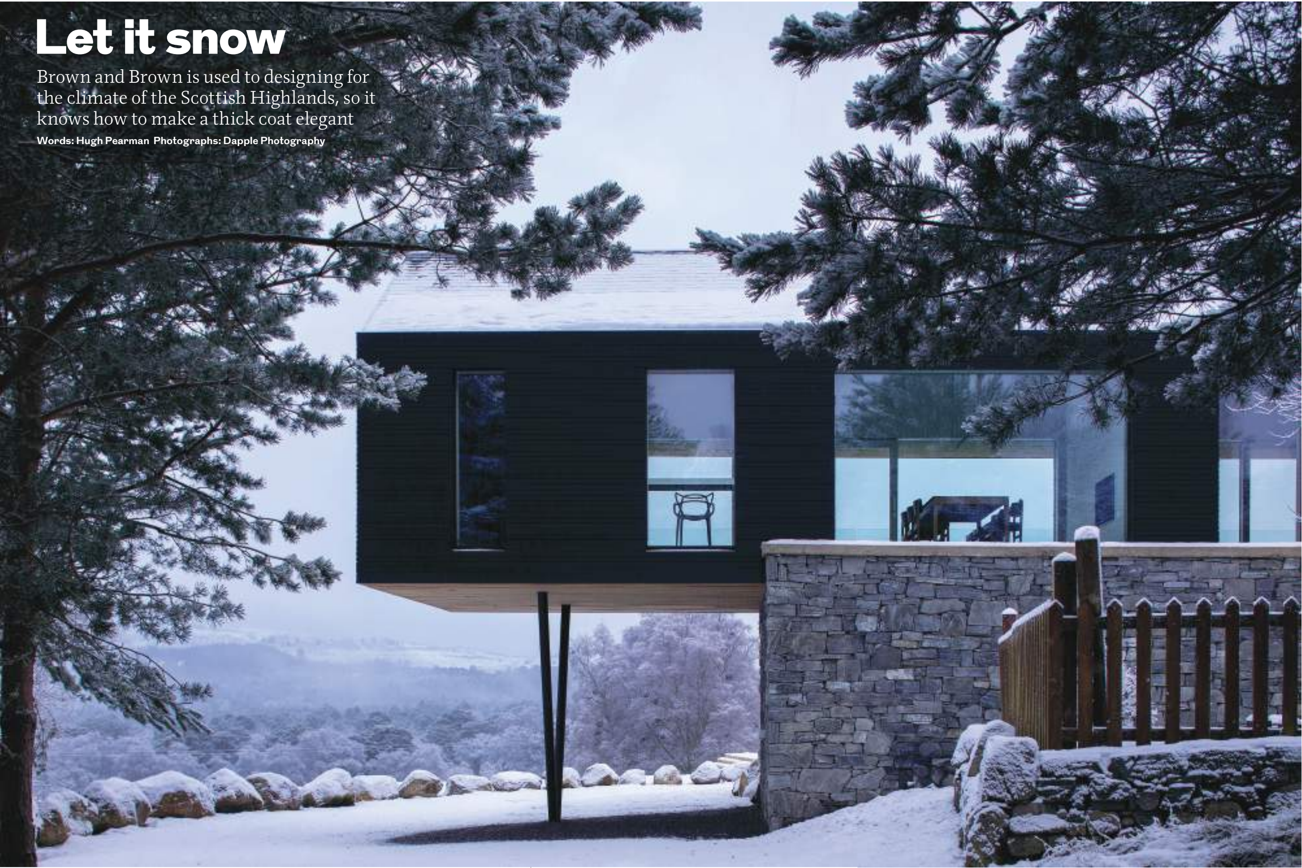
Right and left The new extension continues the ground floor of the original farmhouse over the sloping side onto a new plinth that ends with a cantilever.
