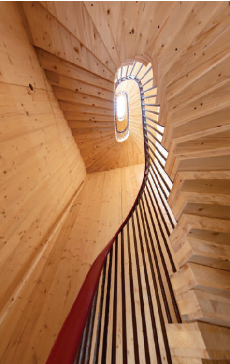
Above The sculpted soffit celebrates the fact that each tread is comprised of two mechanically connected CLT pieces. Above right The connection methodology of the staircase to the timber walls.
