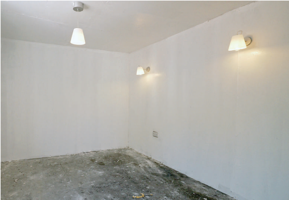
Top A structural engineer finds the fire wall cold to the touch. Above One of the burnt rooms rapidly and fully restored and ready for occupation. Removal and replacement of burnt plasterboard and replacement of electric fittings took about 2 hours and 40 minutes. Right Inside one of the rooms before the test was started.
