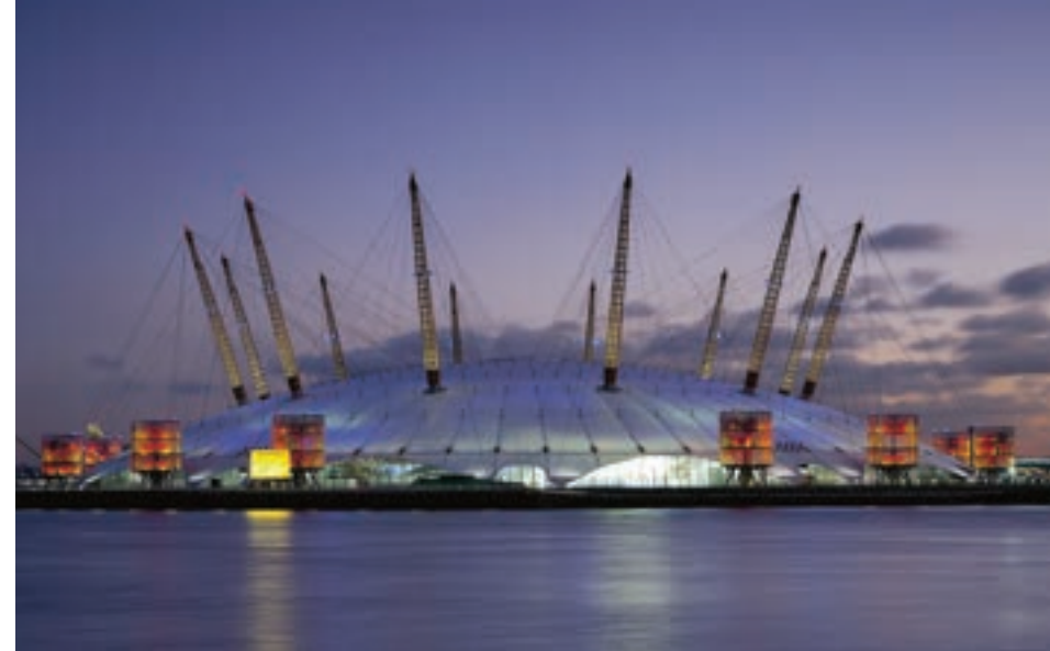
Right The Millennium Dome was completed in 1999 for £42 million. Its 320m diameter roof weighs less than the air contained within.
