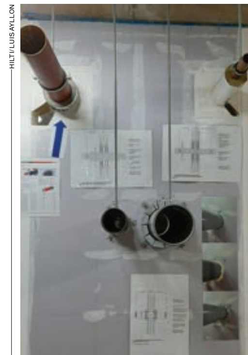
Above A control installation was set up on site at the MMUH so firestop installers could check the precise installation procedures for each application.
