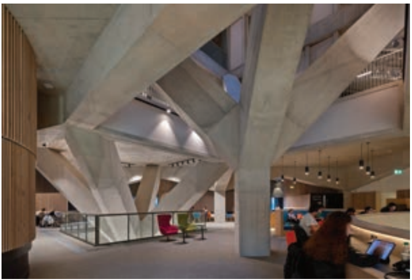
Below Developed with AKT II, the structure twists and twists again to create the 20m, 15.2m, 10.8m and 7.6m grid.
