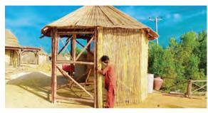
Above from top The process of building skills and making shelters starts with marking out the space on the ground; the bamboo frames are made; local women make the matting; finally the matting is attached to the frame.
