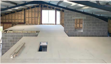
**Above** The first floor deck is formed using West Fraser CaberDek.
