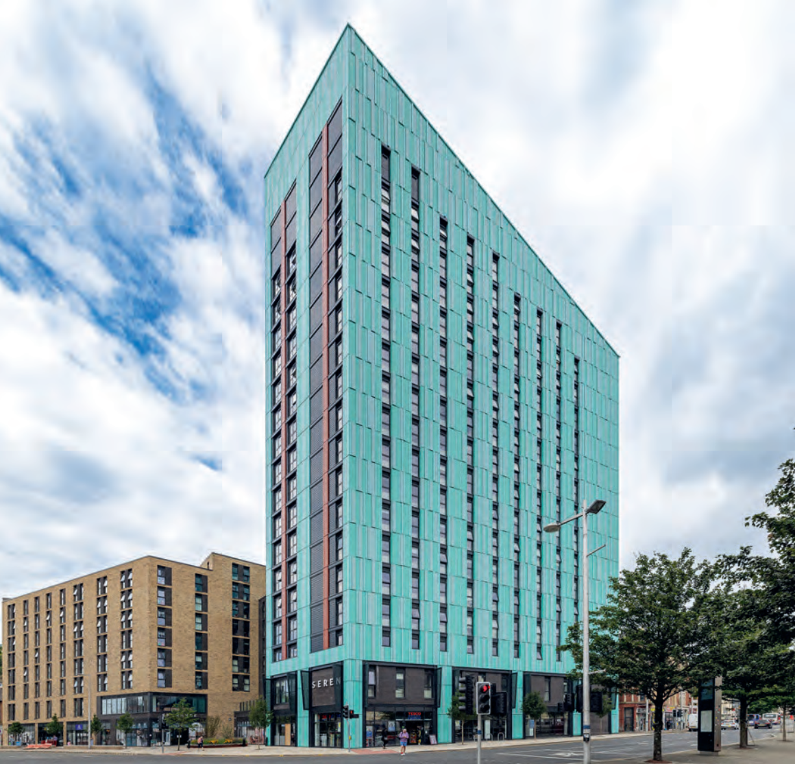
Left Anvil pressed plank secret fix system on Seren student accommodation in Swansea.
