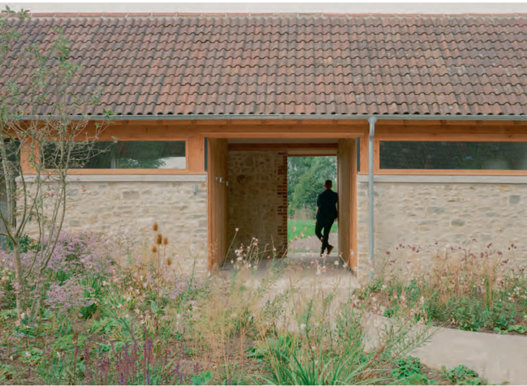
Above A passage through the northern range leads to the boardwalk. Walls reconstructed in timber are less deep, allowing better turning circles for wheelchairs within. Right Kitchen worktops with hob and sink can be lowered electrically.
