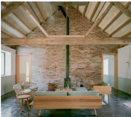
Above Plywood soffits sit above original trusses, repaired and retained where possible. Below left High contrast between floors and walls, or window frames and handles, helps guests with visual impairment. 1 Church 2 Biomass boiler 3 Dutch barn 4 Farmyard 5 Workshop 6 Water treatment 7 Bike/wheelchair store 8 Parking 9 Community space 10 Cottage 11 Breezeway 12 Courtyard 13 Boardwalk
